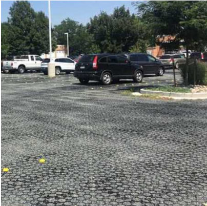
True Grid permeable paving & gravel to carpark
